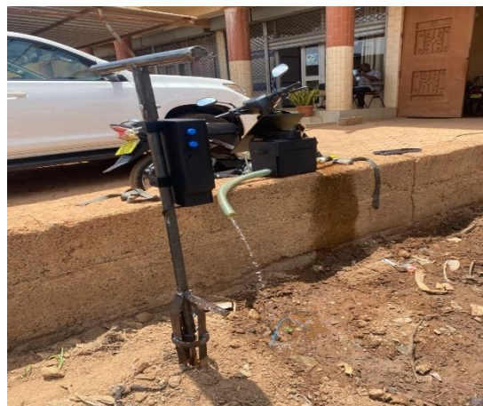
Figure 35: Experimental Test of the Smart Irrigation System Demonstrating Water Flow through the Trigger
