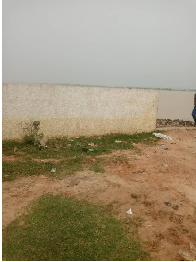
Plate III: Retention wall to prevent the Niger river overflowing its banks at Lokoja, source (field work, August 23, 2023)
