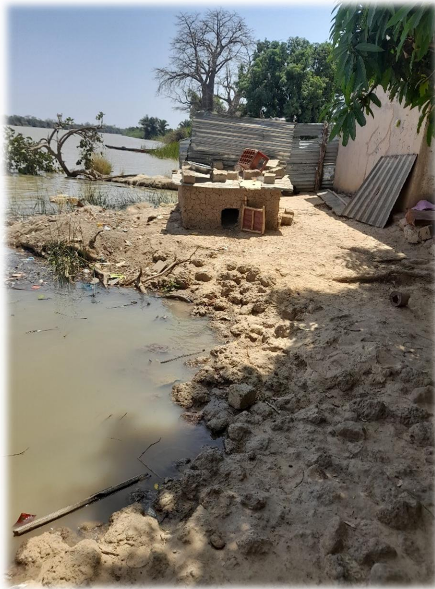
Figure 7: Example of river encroachment of less than a meter to houses in Kuntaur Wharf Town-CRR North (author's own, March 2023)
