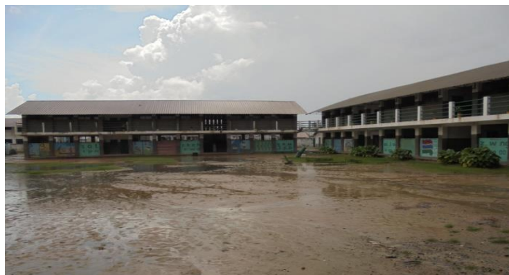
Figure 7: Inundated school compound
