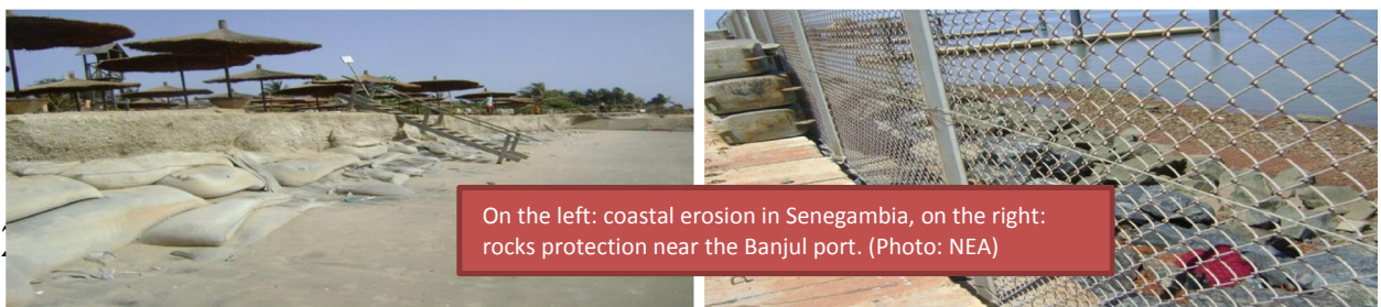
Photo 1.1 Coastal erosion at Senegambia and Banjul port
