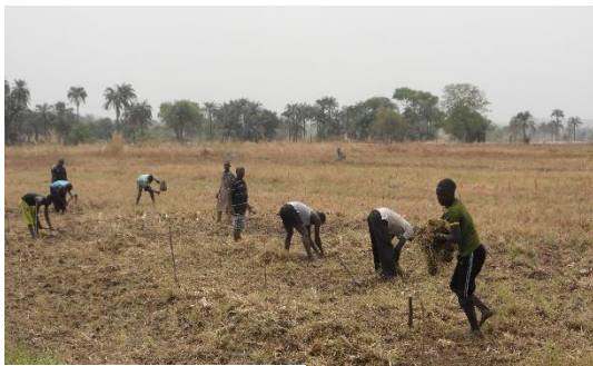
a) Land grading and levelling
